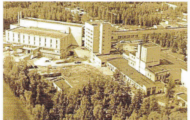
Top view of IBR-2 reactor building
