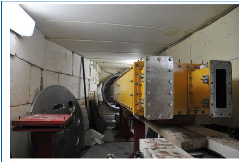
Fig. 12. The head part of the mirror neutron guide installed on beam 6 of the IBR-2 reactor in the framework of the realization of the project of construction of the new DN-6 diffractometer for microsample investigations.
