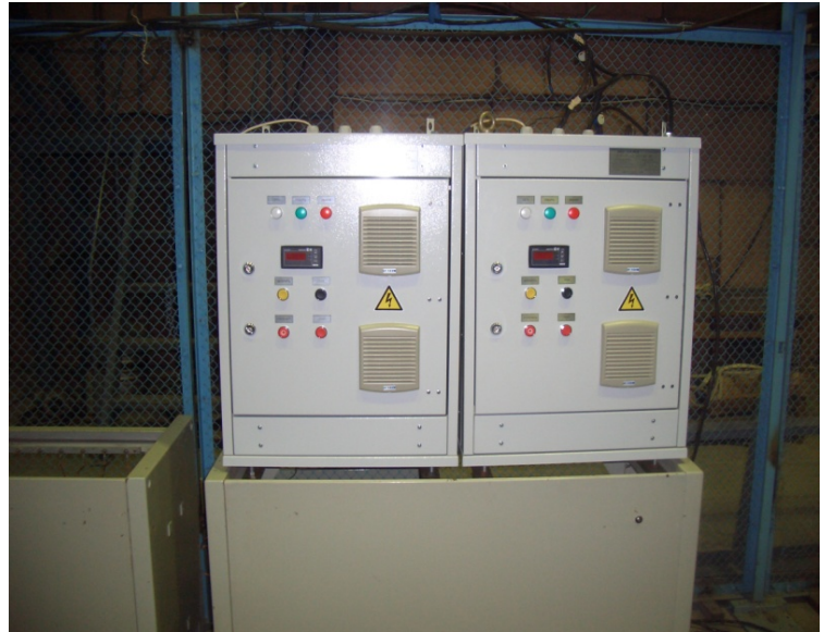
Fig. 10. An electric drive from Toshiba (22 kW) for a background chopper (left) and two electric drives (2.2 kW) for \lambda -choppers (right).
