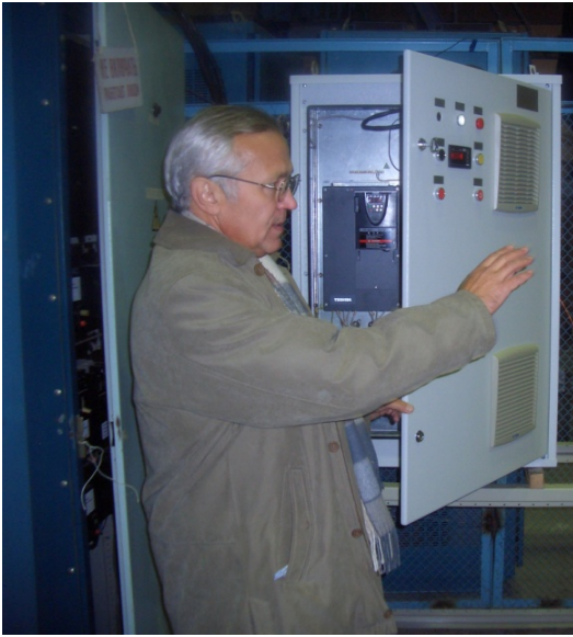
Fig. 10. An electric drive from Toshiba (22 kW) for a background chopper (left) and two electric drives (2.2 kW) for \lambda -choppers (right).
