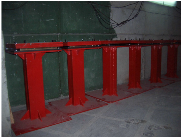
Fig. 7. The beam-positioning support pillars of the neutron guide head part of beam 7.
