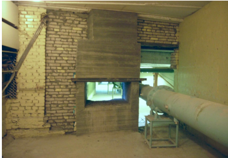
Fig. 6. Reconstruction of the supporting column in bldg.117 for laying curved neutron guides for the EPSILON and SKAT spectrometers.
